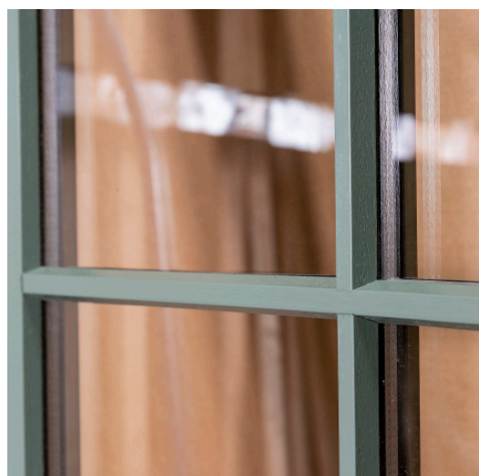
Astragal bars over internal spacers
